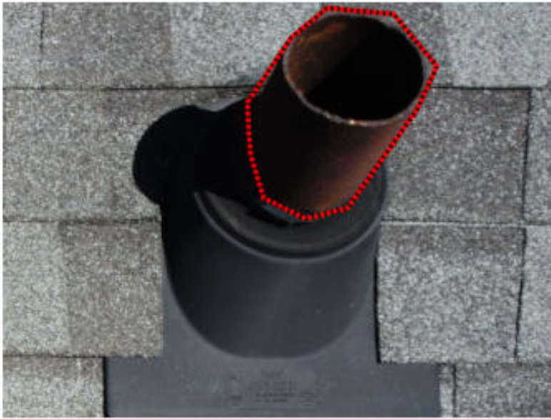
DETAILED VIEW - PENETRATIONS #1
