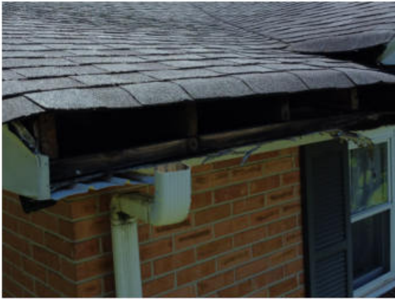
DETAILED VIEW - GUTTERS AND DOWNSPOUTS #1
