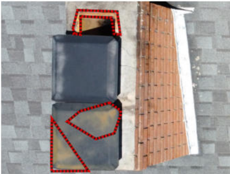
DETAILED VIEW - PENETRATIONS #3
